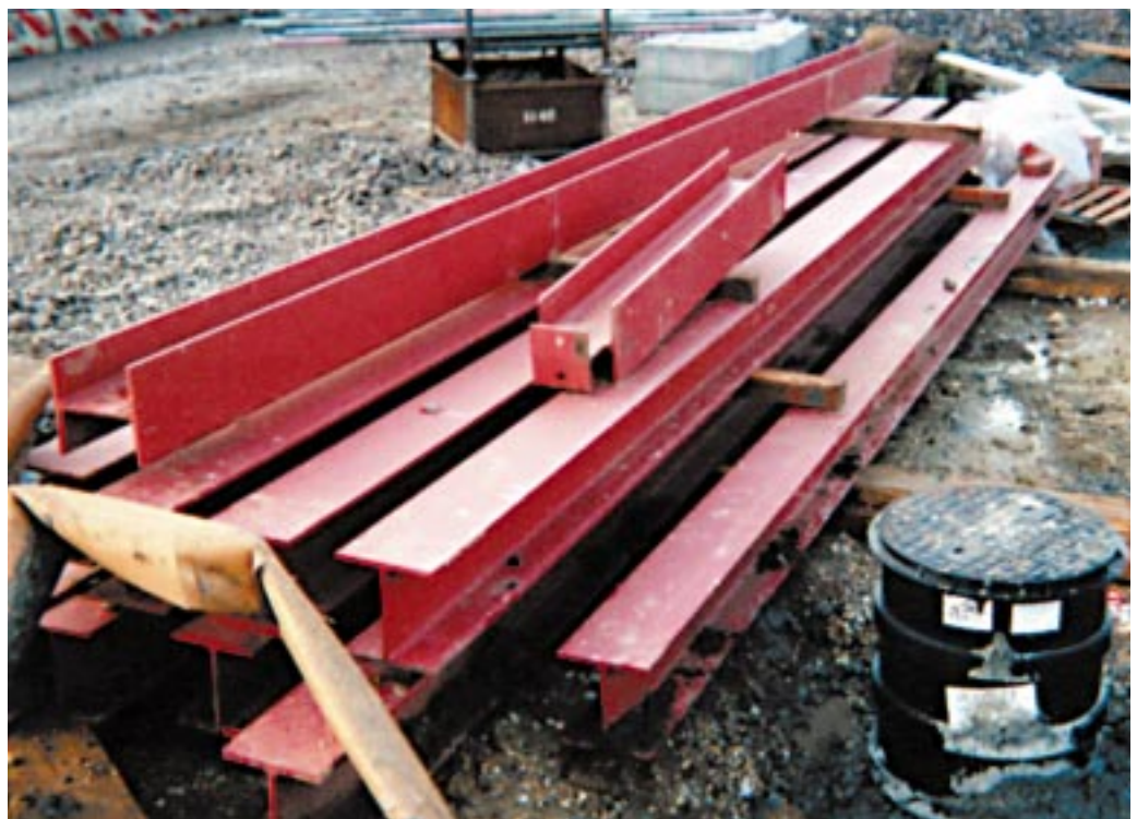
All the structural steel is reclaimed
