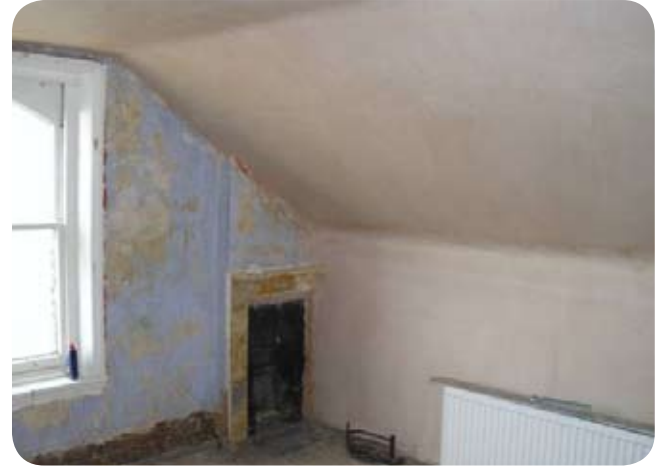
After: Fully insulated rafters with plaster board covering.
