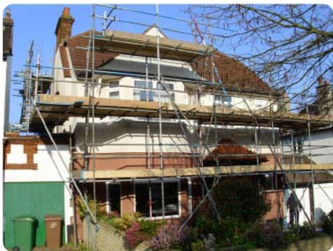
Installing external insulation: Step 1: scaffolding erected.
